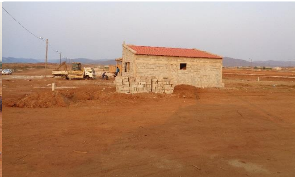
Housing construction at the Cabrais settlement
