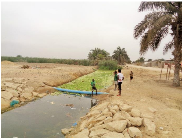
A drainage that had overflowed due to the piled up garbage in Catumbela
