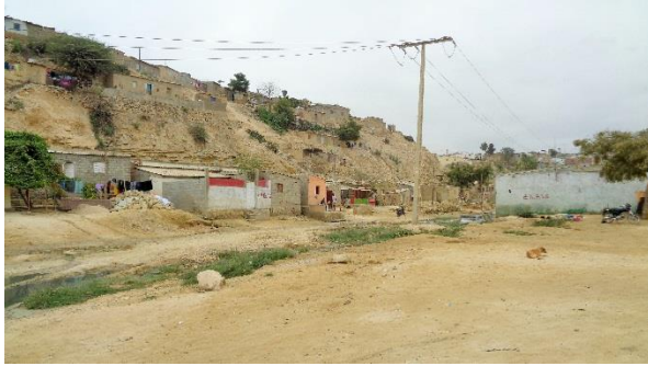
The houses affected by the flood in Lobito
