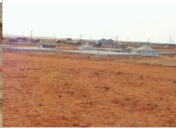
The foundations for the future homes at the Cabrais new settlement
